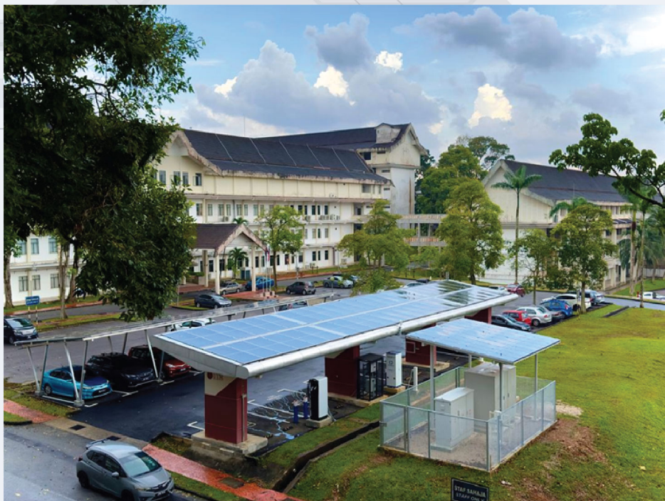
EV Charging Station with BESS at Faculty of Electrical Engineering, UTM
