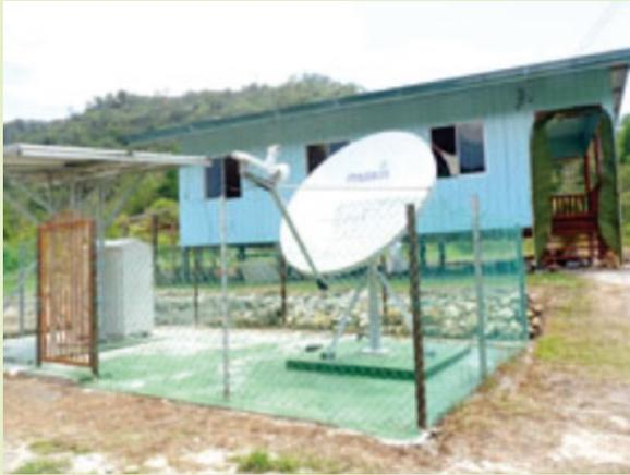
*Solar powered telecommunication system (VSAT) in Sarawak*
